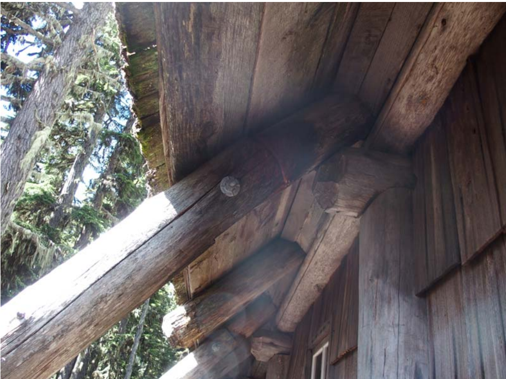
Figure 16. Tilly Jane Ski Warming Hut. View of previously-spliced buttress/rafter situated on south elevation. USFS digital photograph obtained 07/18/2016 by Michael D. Dryden.
