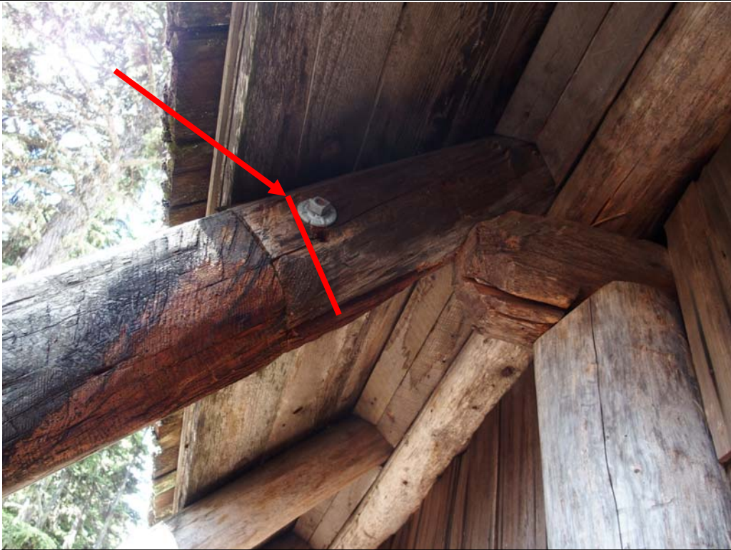
Figure 21. Close-up view of previously spliced buttress/rafter on south elevation. The location of the current splice tends to wick moisture up into the splice. The new splice would be situated 2" to 3" higher under the eave to be more protected. Red arrow points to the proposed splice location. USFS digital photograph obtained 07/18/2016.
