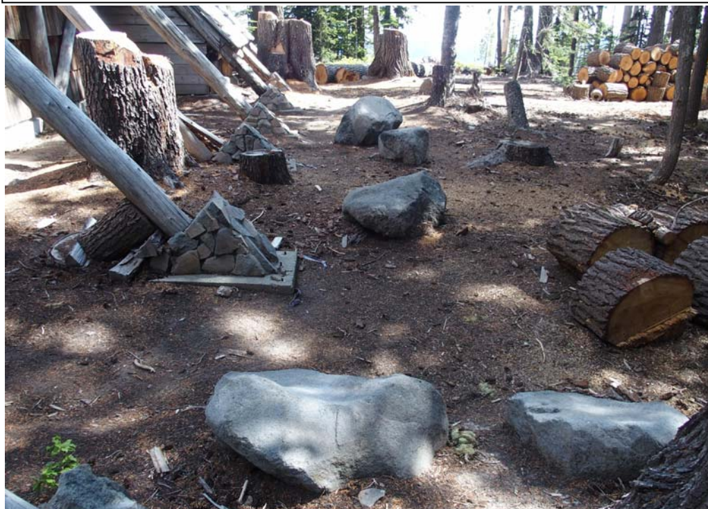
Figure 14. Tilly Jane Ski Warming Hut. View of buttress/rafters and boulder anchors replaced on south elevation. View looking east. The previous boulder anchors lie just to the right of the buttress/rafters. USFS digital photograph obtained 07/18/2016 by Michael D. Dryden 07/18/2016.
