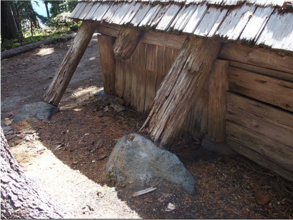
Figure 17. Tilly Jane Ski Warming Hut. View of intact original buttress/rafter boulder anchors. USFS digital photograph obtained 07/18/2016 by Michael D. Dryden.
