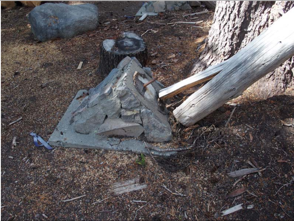
Figure 15. Tilly Jane Ski Warming Hut. Close-up view of concrete buttress/rafter anchor replacement with masonry veneer. USFS digital photograph obtained 07/18/2016.
