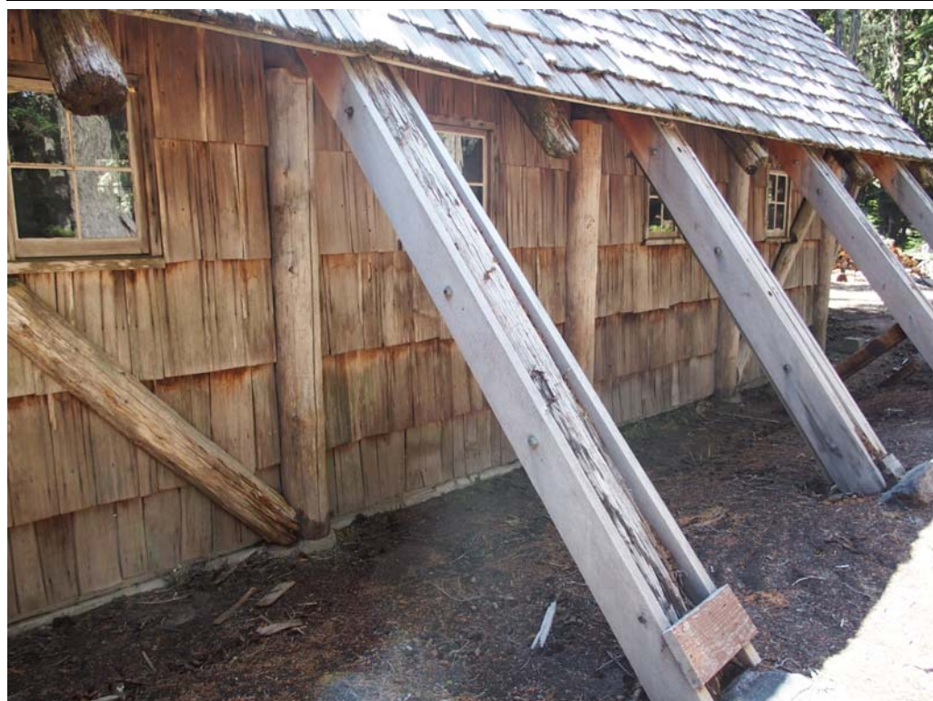
Figure 10. Tilly Jane Ski Warming Hut. Photograph of deteriorated buttress/rafters on north elevation "sandwiched" between 2"x10" boards. USFS digital photograph obtained by Michael D. Dryden 07/18/2016.
