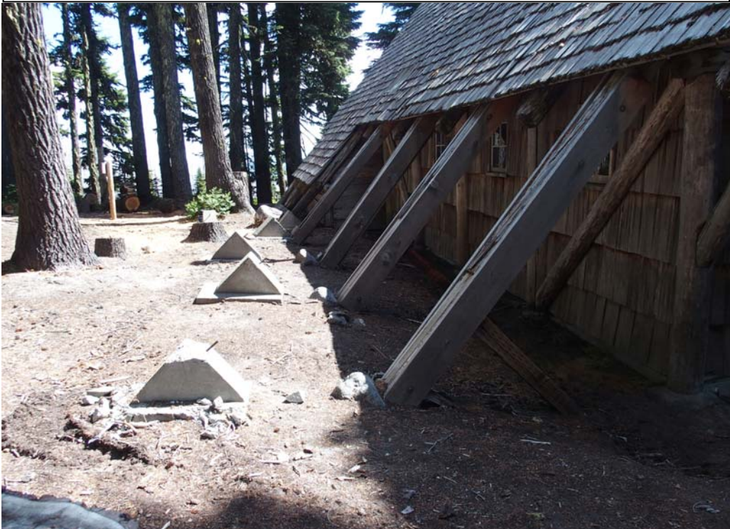
Figure 12. Tilly Jane Ski Warming Hut. Overview of rafter/buttresses on north side, view looking east. Concrete forms intended to replace boulder anchors situated to left of buttress/rafters. USFS digital photograph obtained 07/18/2016.
