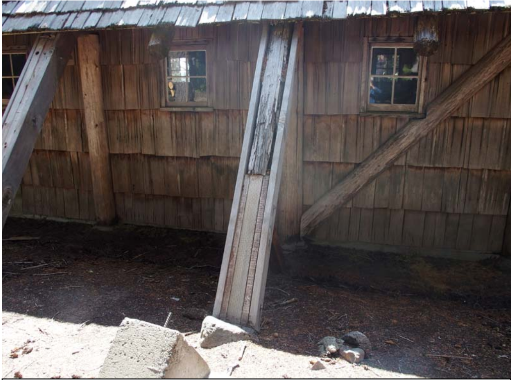
Figure 11. Tilly Jane Ski Warming Hut. Close-up view of deteriorated buttress/rafters on north side of structure with augmented timbers. USFS digital photograph obtained 07/18/2016
