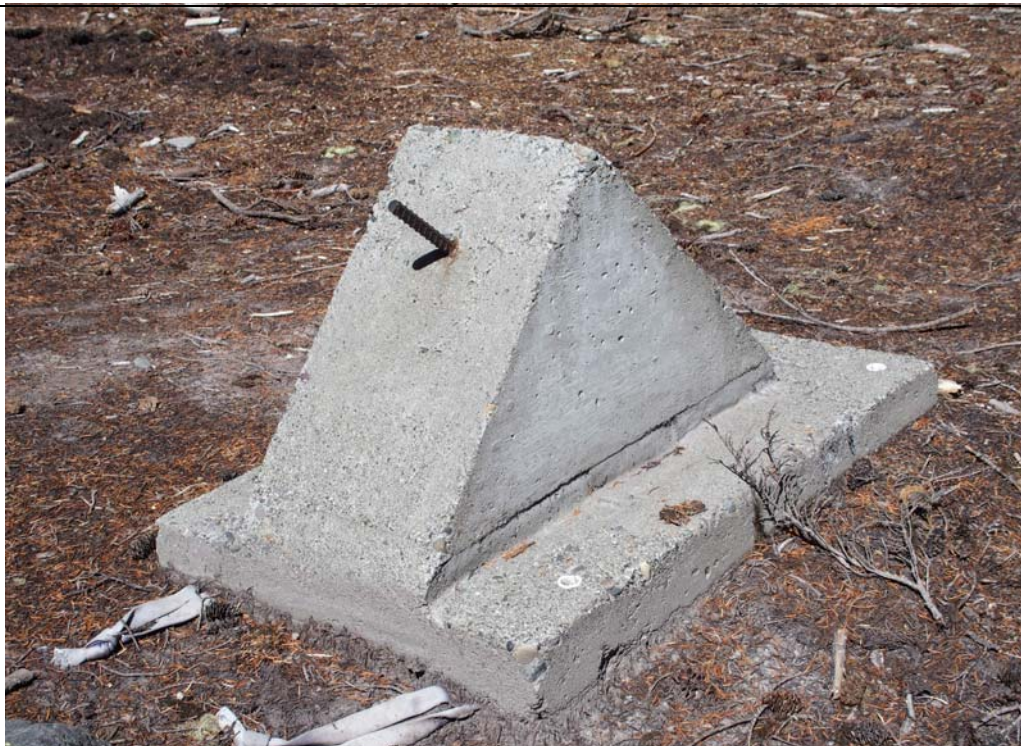
Figure 13. Tilly Jane Ski Warming Hut. Close-up view of concrete form intended to replace boulder buttress/rafter anchors. USFS digital photograph obtained 07/18/2016 by Michael D. Dryden.
